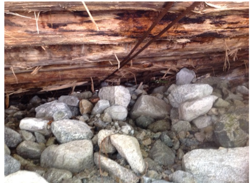
looking through from outlet
